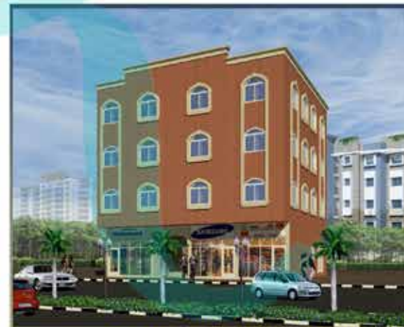
G+3 BUILDING, MUWEILAH, SHARJAH
